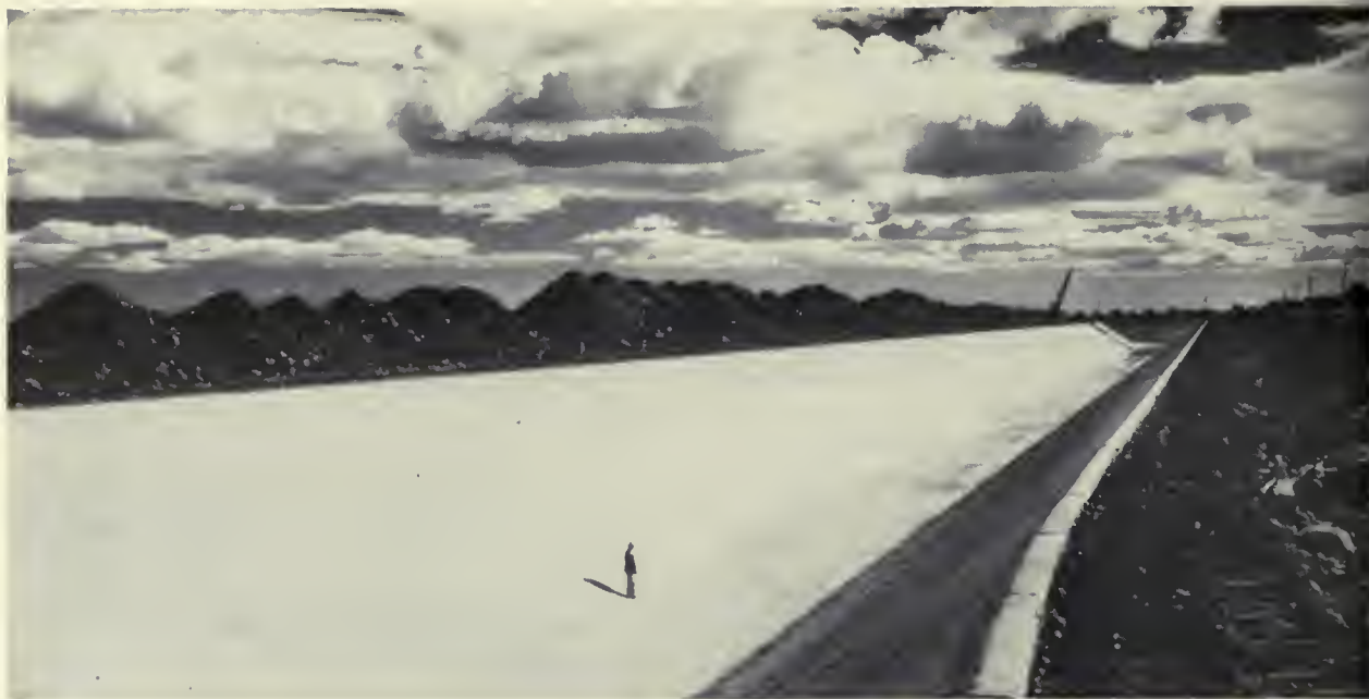
MAIN ARTERY for Irrigation Block 40 in Grant County, Washington, is East Low Canal, above. Photo by H. E. Foss, Region 1.
